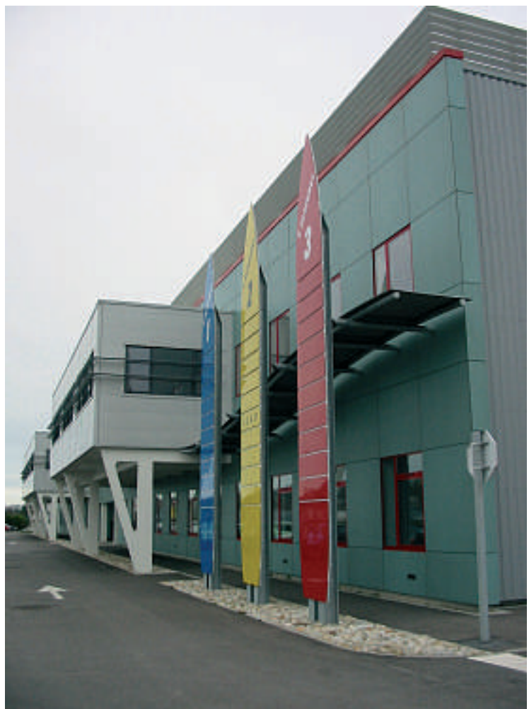
Building E. Placenet, Saint-Martin-Boulogne (France) BET: Maning
