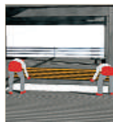
Laying of the floor decks
