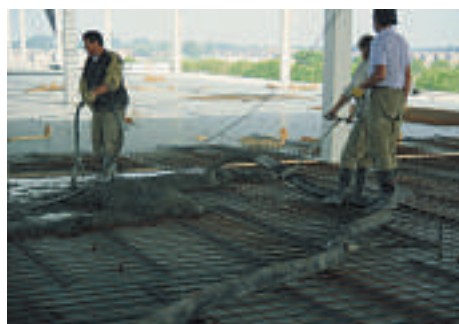
On site concrete pouring of the slab
