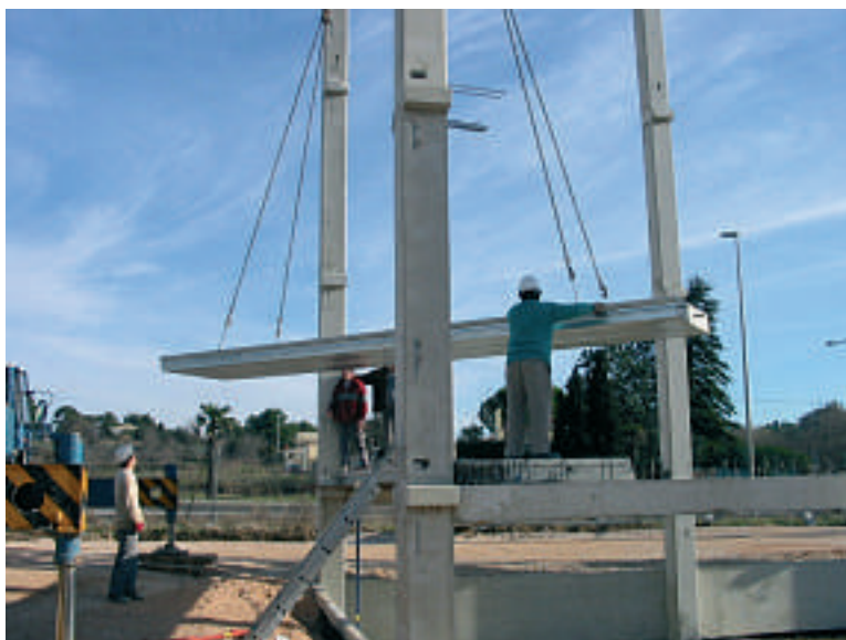
Installation of a prefabricated floor
