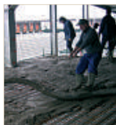
Pouring of concrete
