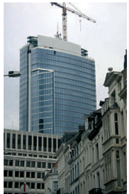
Tour Madou, Brussels (Belgium) ARCHITECTS: Assar/archi 2000
